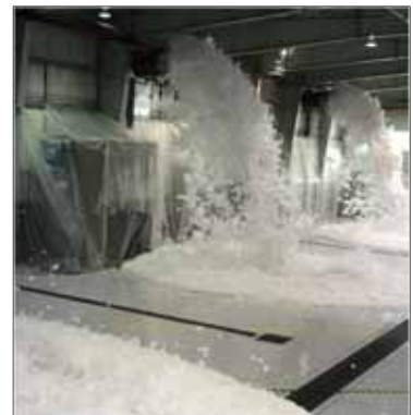
Example of hangar fire suppression system being tested
