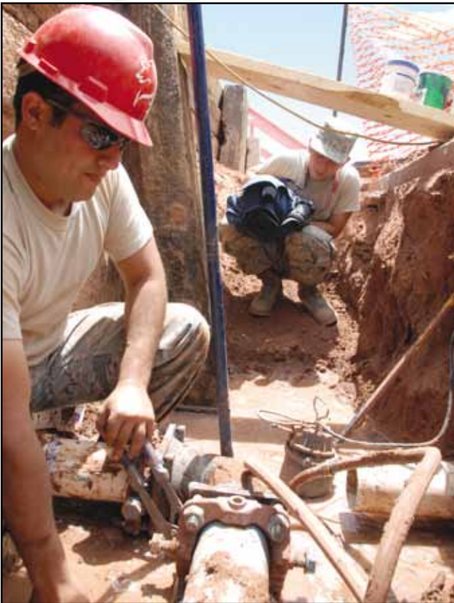
Staff Sgt. Joseph Bonamico, 201st RHS, Det. 1, connects a 90 degree pipe fitting in an effort to repair a faulty water line while Senior Airman Thomas Grimes, 111th FW, captures video of the muddy work.
