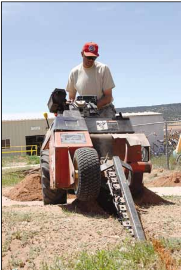
Senior Master Sgt. James Gray, 201st RHS, Det. 1, digs a trench for underground cable as part of the new nurse's station project.
