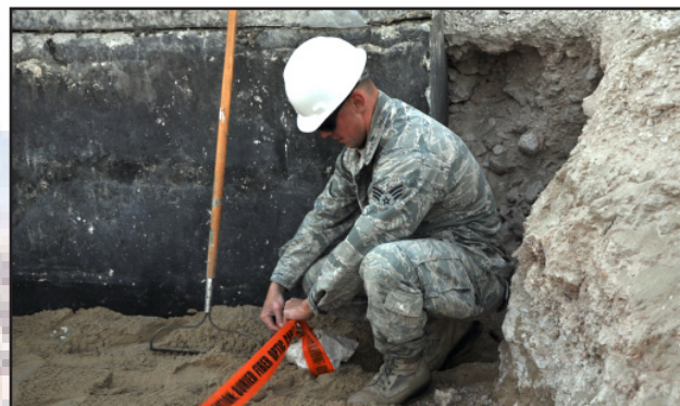
Airman 1st Class Christian Blaydon (shown left) and Senior Airman Mark Wojdylo (shown above), A67 Engineer and Installation team members deployed from the 270th Engineering Installation Squadron, Pennsylvania Air National Guard, lay down and secure warning tape over sand that covers a newly replaced ground tactical fiber run at an undisclosed location in Southwest Asia on Dec. 19.
