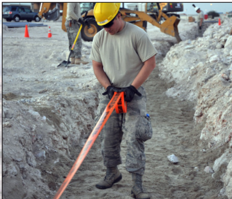
Airman 1st Class Christian Blaydon (shown left) and Senior Airman Mark Wojdylo (shown above), A67 Engineer and Installation team members deployed from the 270th Engineering Installation Squadron, Pennsylvania Air National Guard, lay down and secure warning tape over sand that covers a newly replaced ground tactical fiber run at an undisclosed location in Southwest Asia on Dec. 19.
